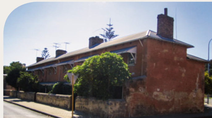
ABOVE Warders' Cottages, Fremantle (1851-1858)
