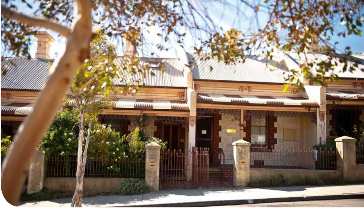
ABOVE: Seven Terrace Houses, Fremantle (1886)
